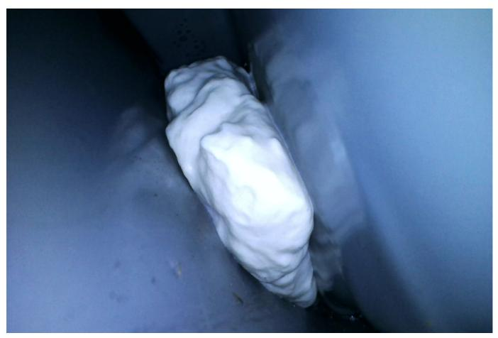
The filler effectively isolates both sides of the lower cavity.
